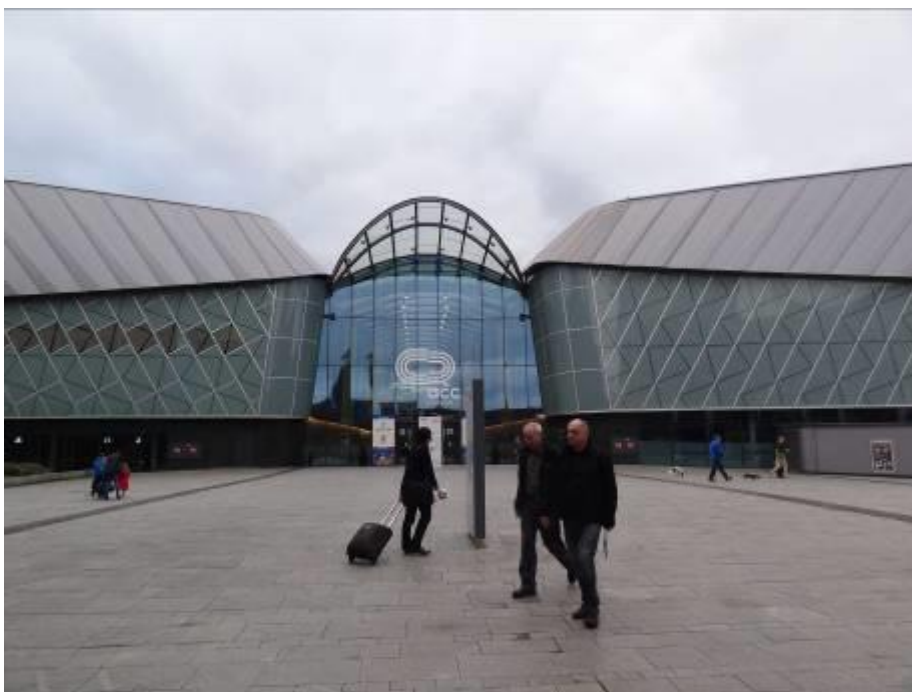
The Arena and Convention Centre (ACC), Liverpool
