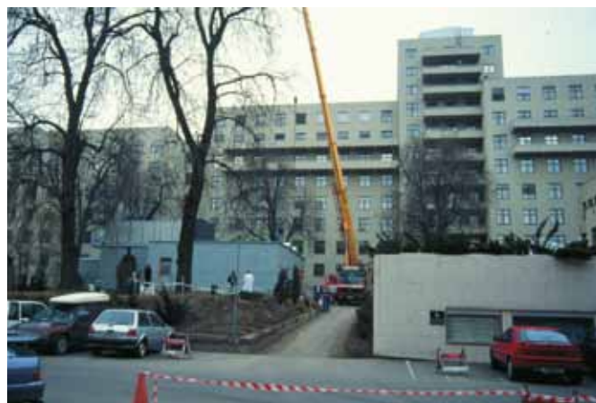
Fig 9-1. The Interventional Signa SP 0.5T MR magnet being hoisted in through the roof of the temporary barracks housing the Intervention Centre at Rikshospitalet in the spring 1996. Courtesy Intervention Centre Oslo Univ Hosp
